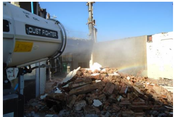
Fig. 6 Example of dust suppression previously used during building demolition.
