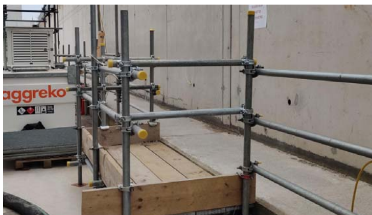
Pictures 11, 12: Passing layby constructed on walkway
