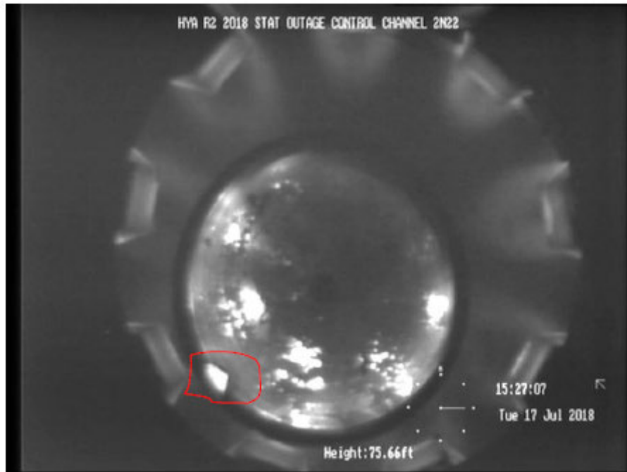
Figure 2: Piece of debris observed in debris pot in control rod channel N22.
