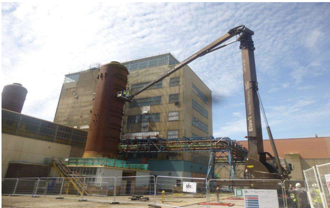
Figure 16: Work on the Reactor 1 heat exchangers.
