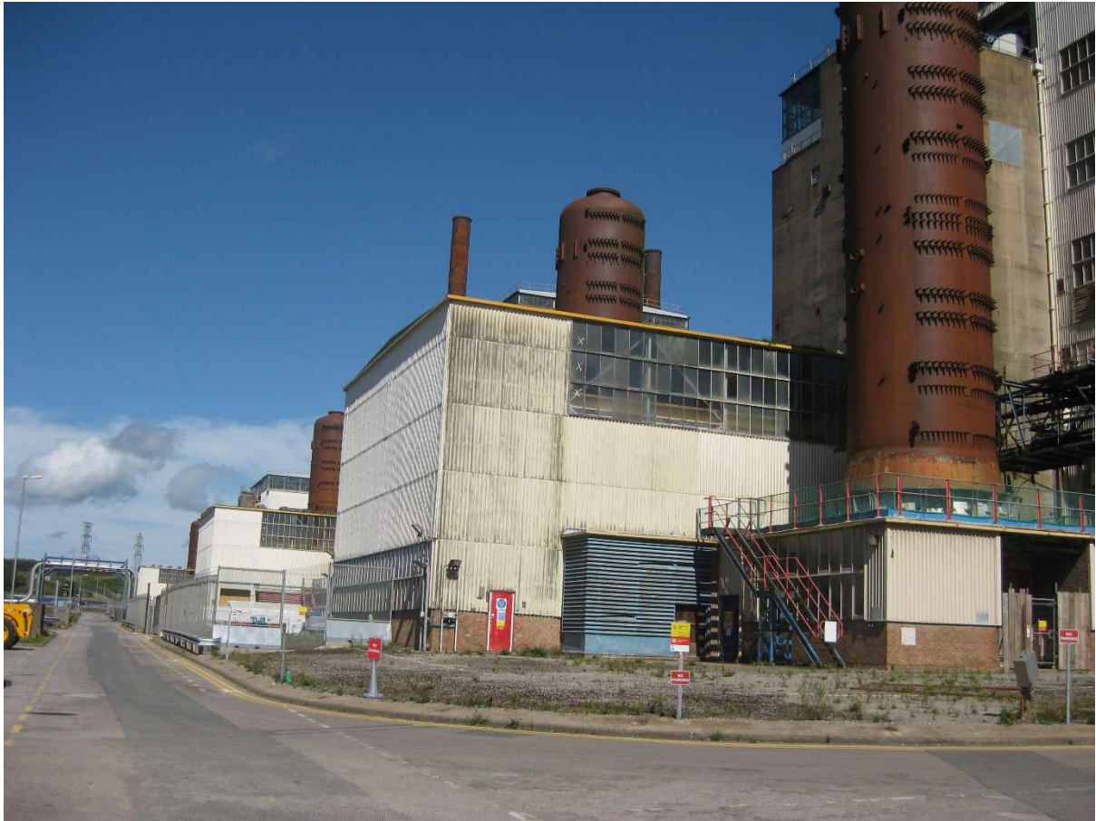
Figure 18: Reactor 2 with Short Blower House to the left.
