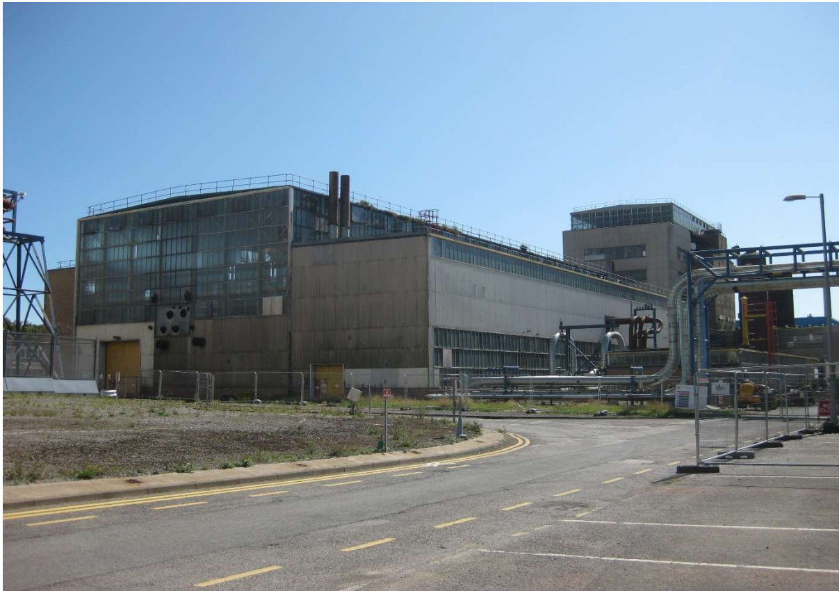
Figure 20: Turbine Hall A.
