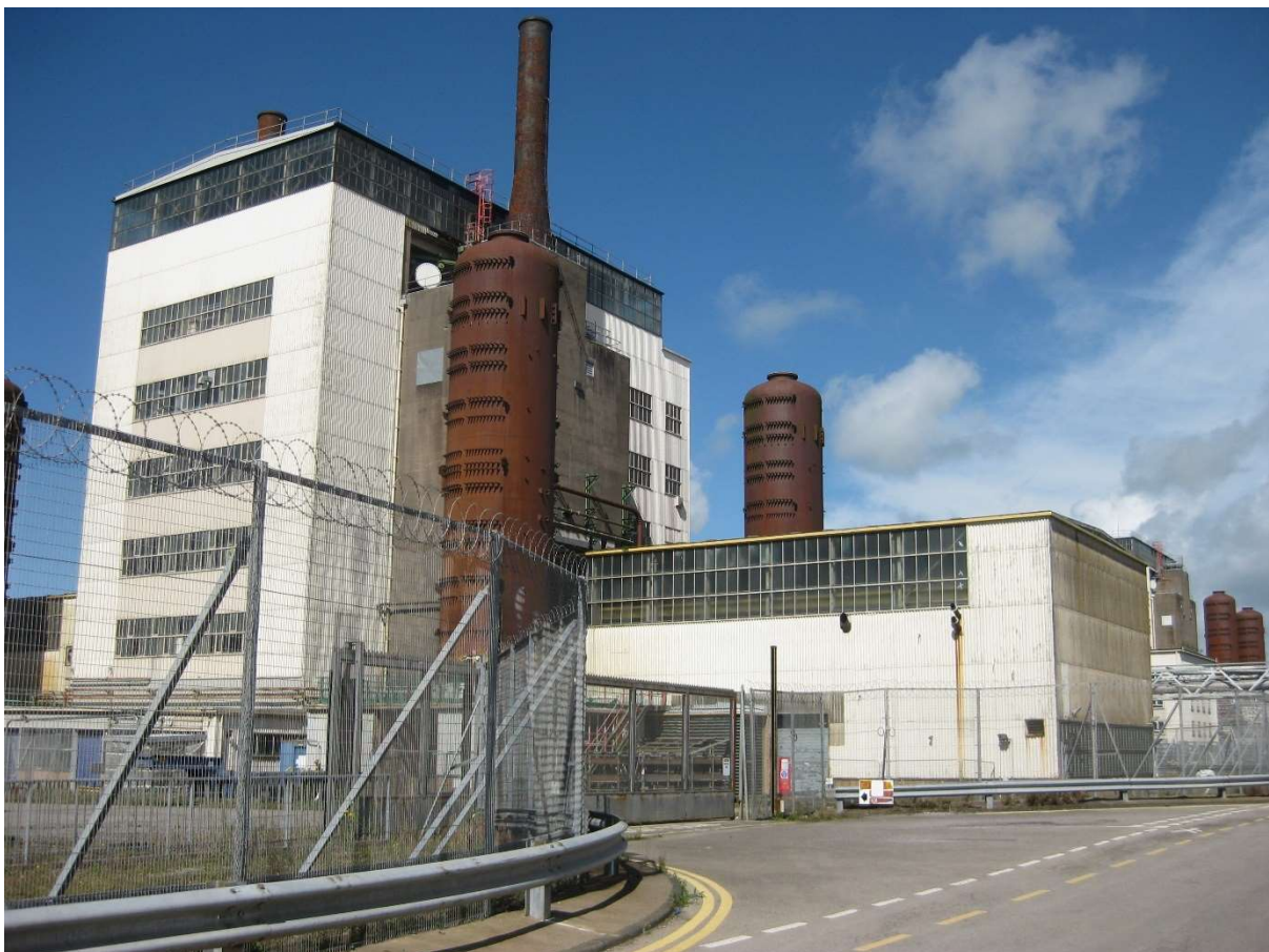
Figure 17: Reactor 3 with Long Blower House to the right.
