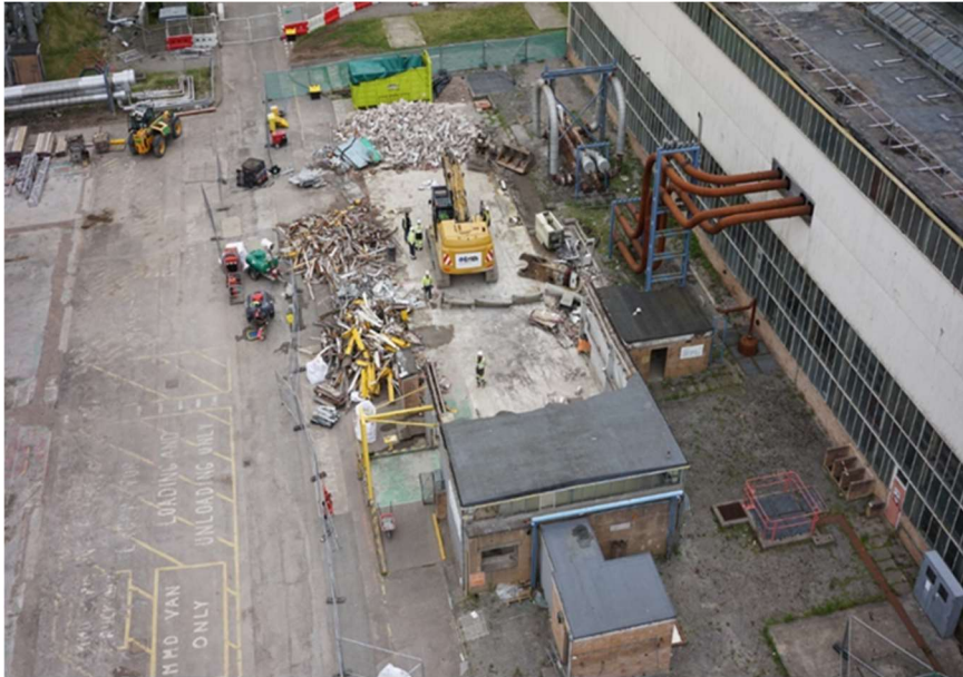
Figure 5: Redundant Control Rod Workshop now demolished to base slab.
