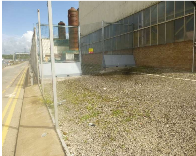
Figure 8: Reactor Compound fence removal after radiological categorisation downgraded to C1/R0.
