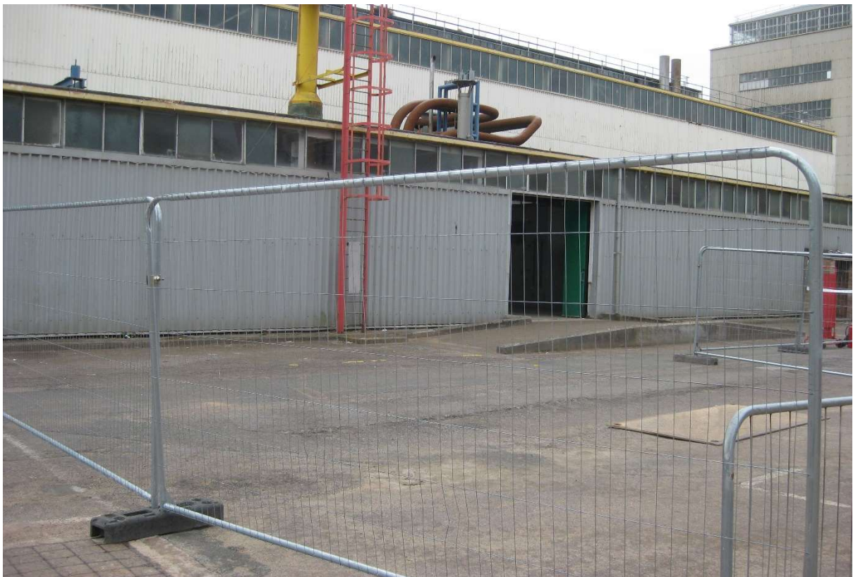
Figure 4: Redundant Control Rod Workshops prior to demolition.
