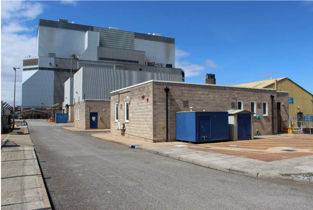
Plate 9. Original ancillary buildings in the eastern site area. View north-west.
