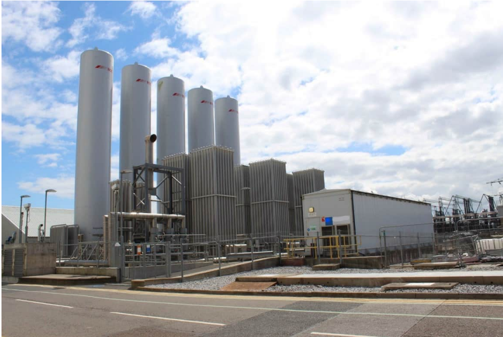
Plate 5. Modern plant to the south of the reactor building. View south-east.
