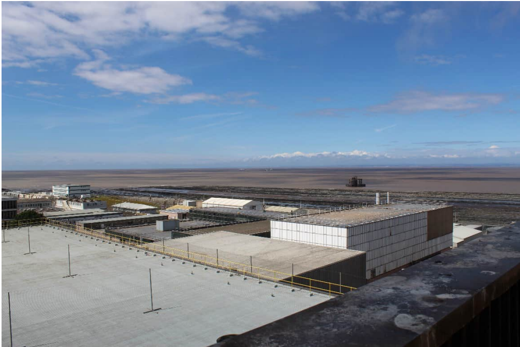
Plate 14. Water intake out to sea to the north. View north-east.
