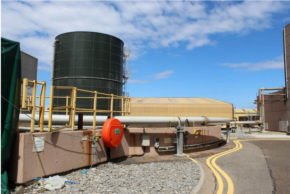
Plate 11. Original and modern ancillary buildings to the north of the turbine hall. View north.
