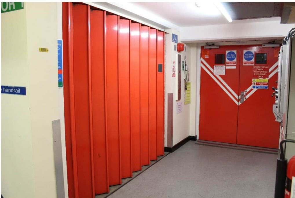
Plate 18. Reactor building interior features.
