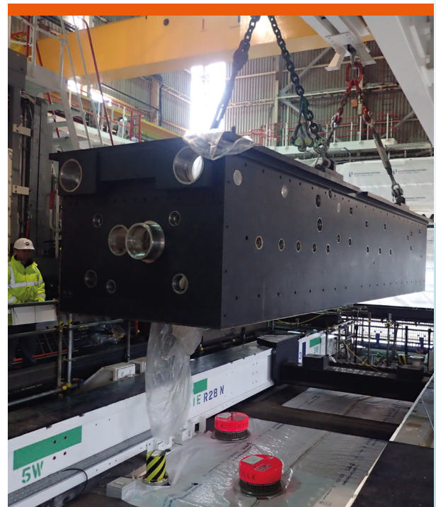
Figure 10: Installation of SEP 1 transfer tunnel
